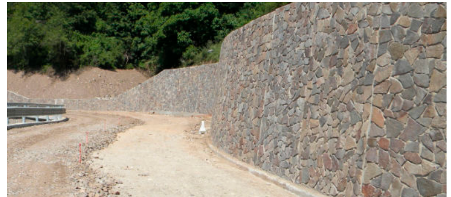
Concrete retaining walls
