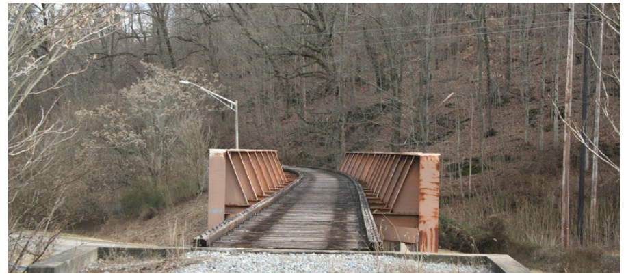
Prefabricated bridge crossings
