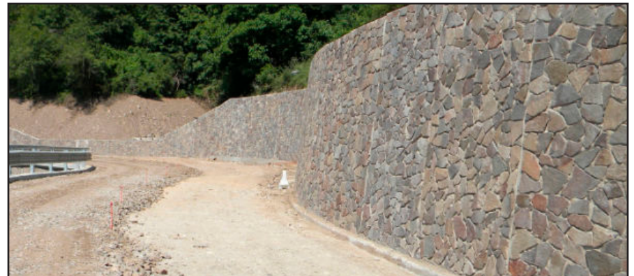
Concrete retaining walls
