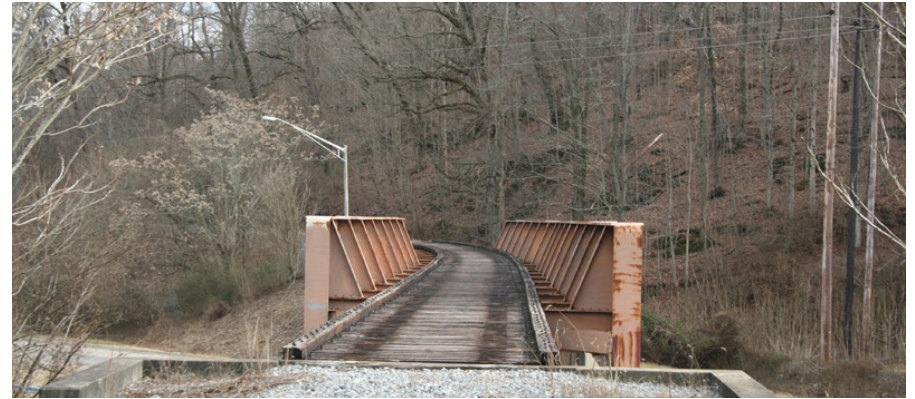
Prefabricated bridge crossings
