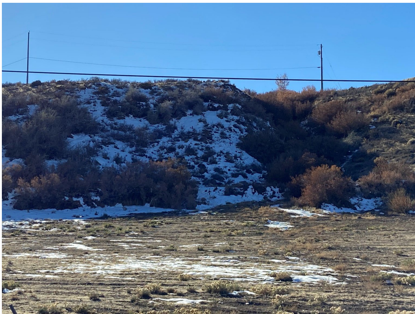
FIGURE 5: Picture of both Olson power poles spanning across the steep riparian drainage (view from Highway 395).
