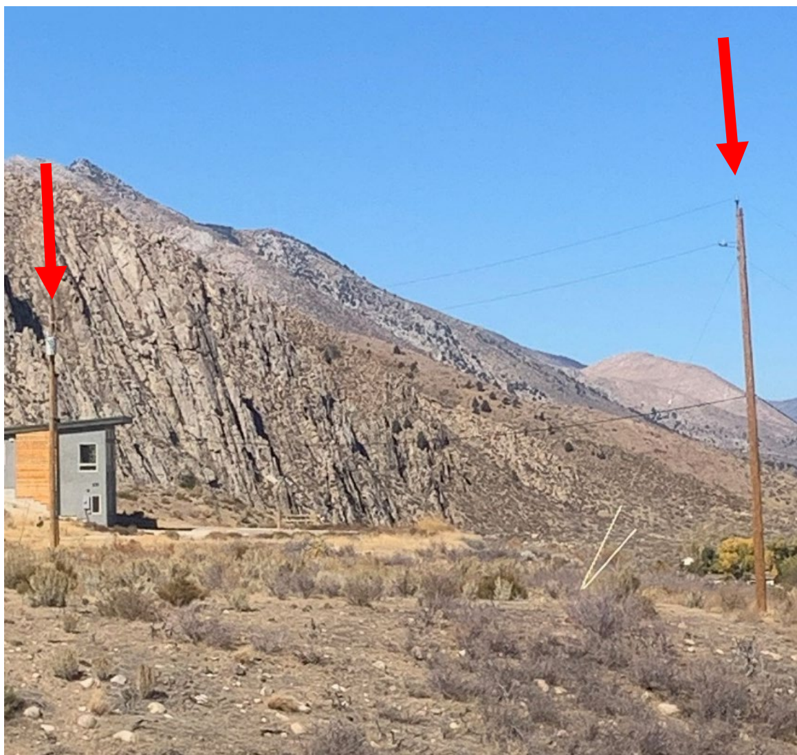
FIGURE 3: Olson Residence showing the two new unauthorized overhead power poles.
