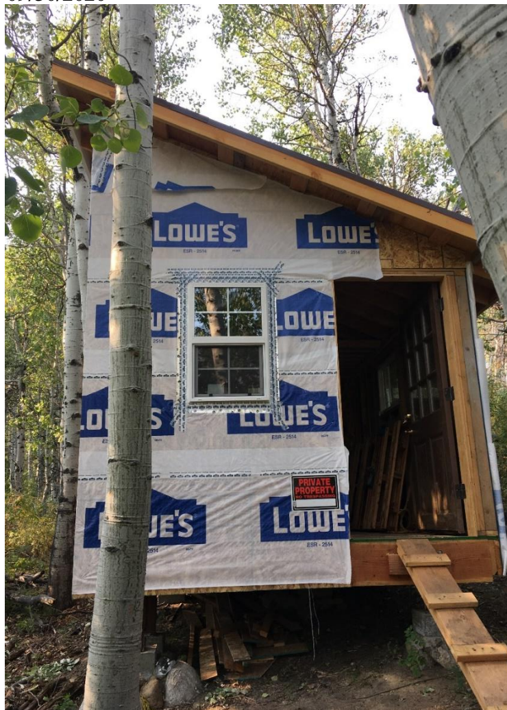
Existing 116-square foot shed, looking west.
