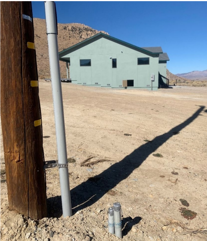
FIGURE 3: Hemminger Residence from the south looking north. Picture shows the last of the 3 poles and then the line is undergrounded the last 100+ feet to the residence.
