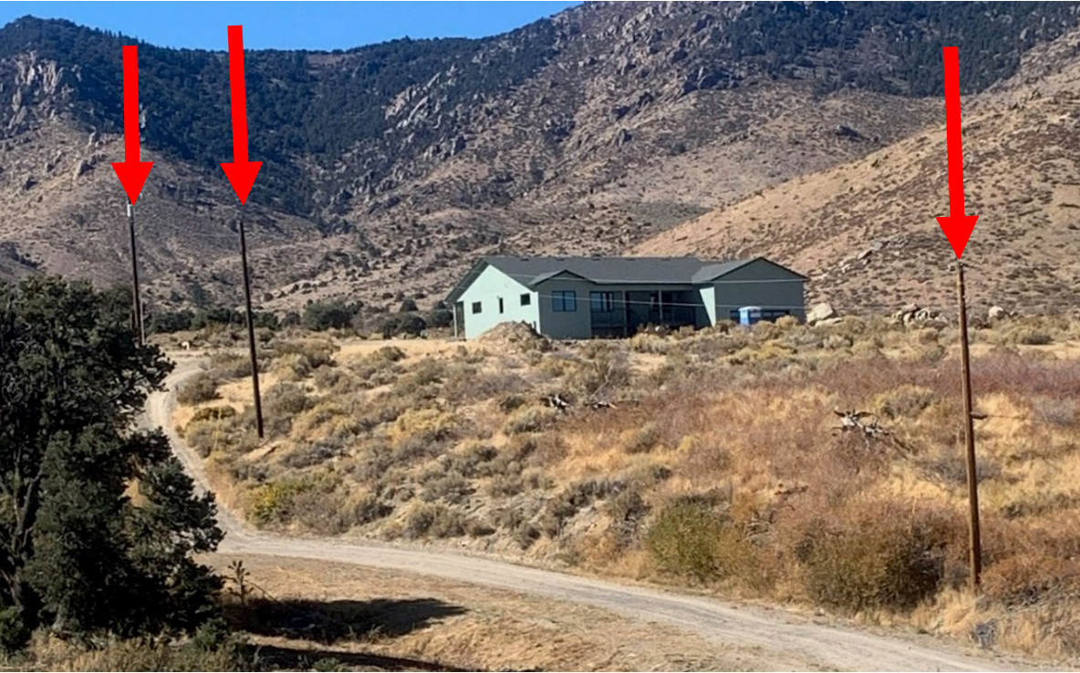
FIGURE 2: Hemminger Residence showing 3 of the 5 new unauthorized overhead power poles.
