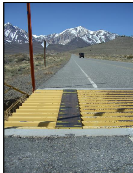
FIGURE 2. Example of Bicycle-friendly Cattle Guard on Benton Crossing Road.
