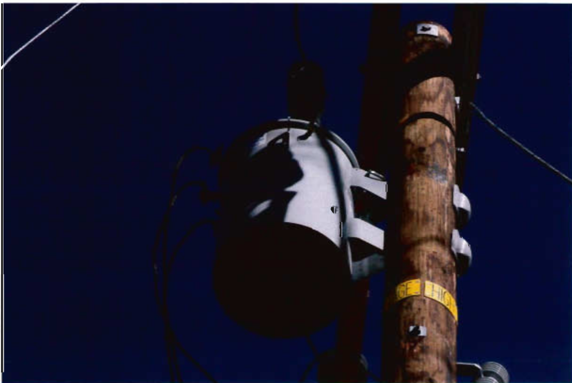
P-KG-176 Close up of transformer and hardware on center of powerpole number 1854107E, facing north
