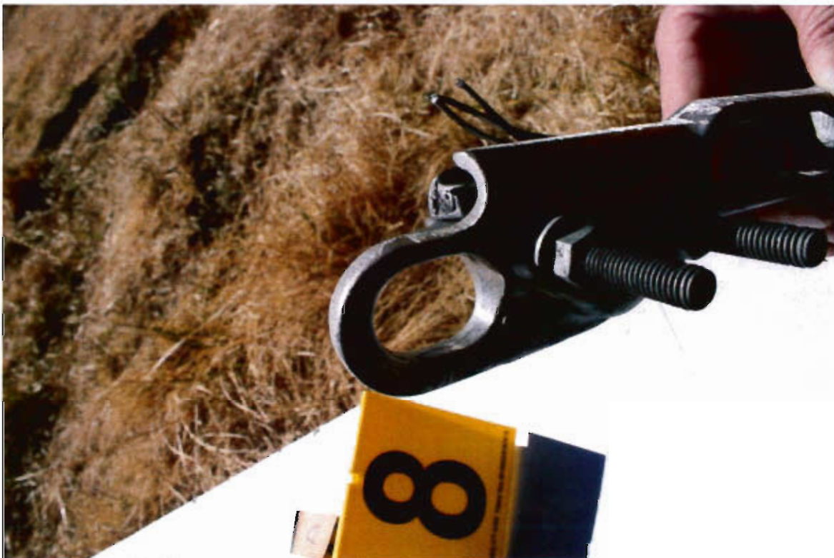
P-KG-284 8a - Close up of wire shoe with piece of power line attached
