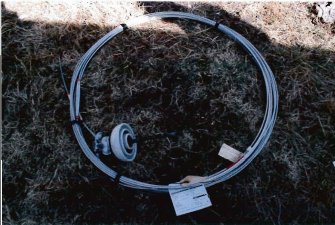
P-KG-386 8d - Collected - Power line section, end 6 and 7
