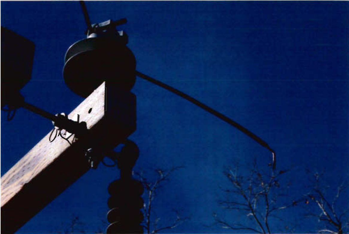
P-KG-267 Close up of hardware on northwest corner of pole number 1854107E from lifted Edison bucket, facing southwest
