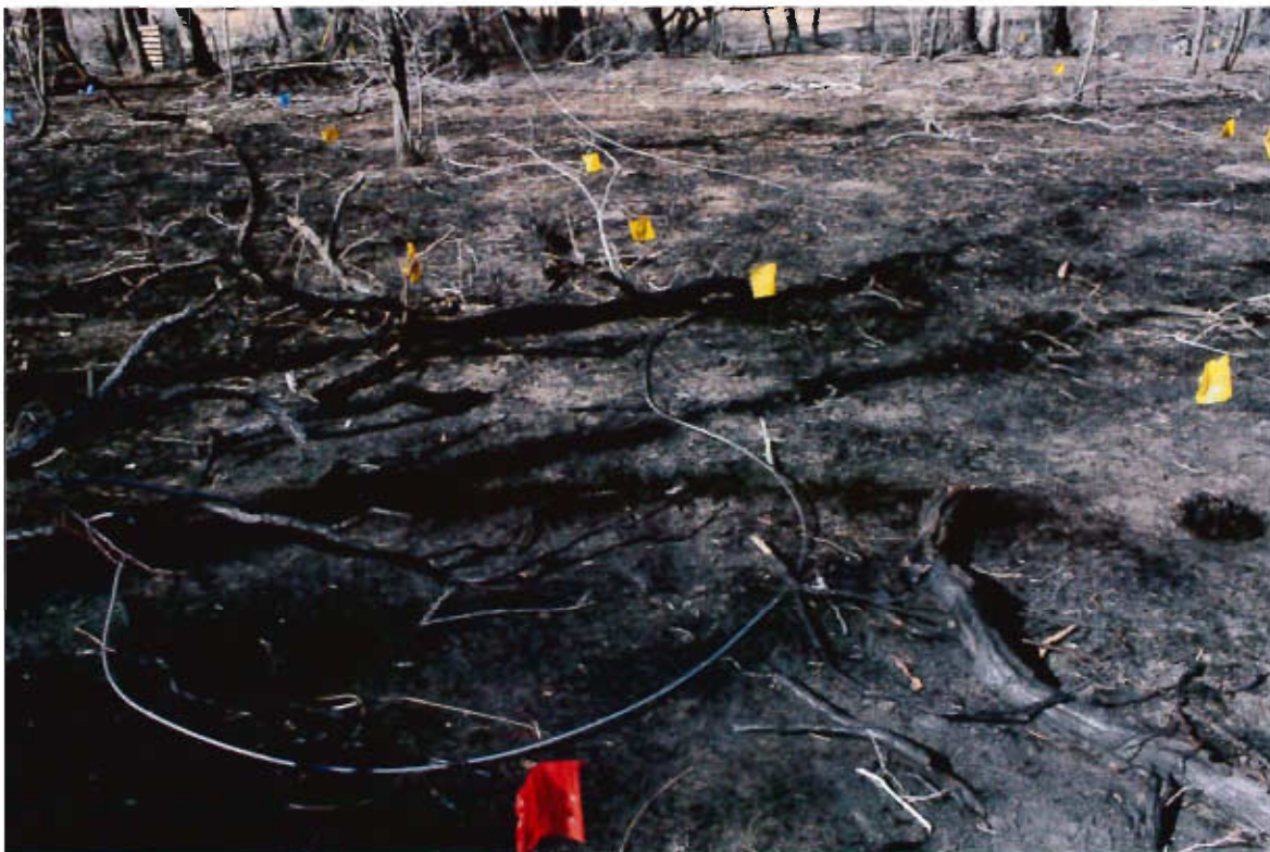
P-KG-184 South powerline, facing west
