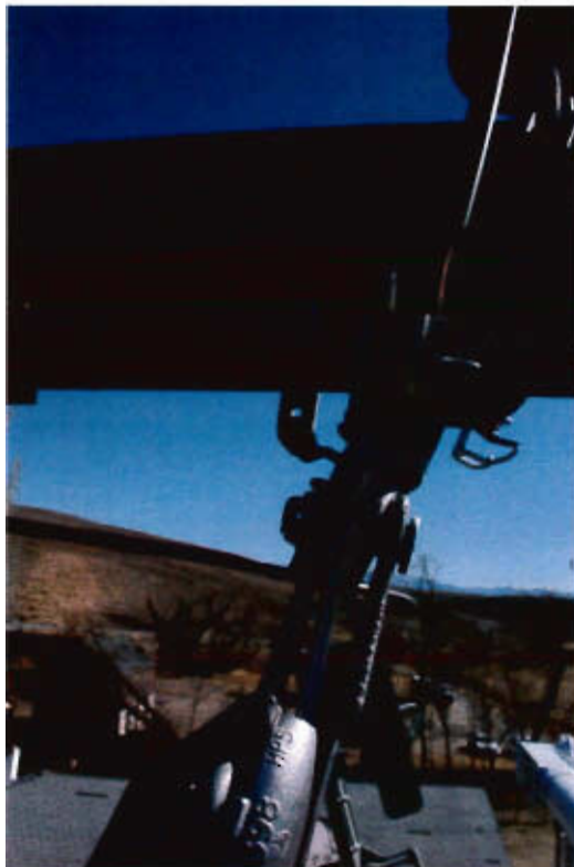
P-KG-275 Close up of hardware on southwest corner of pole number 1854107E from lifted Edison bucket, facing east
