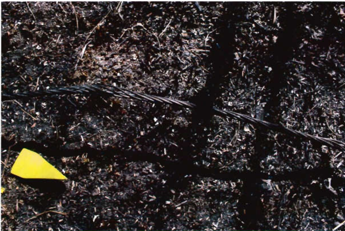
P-KG-340 9b - Power line section close ups from west to east
