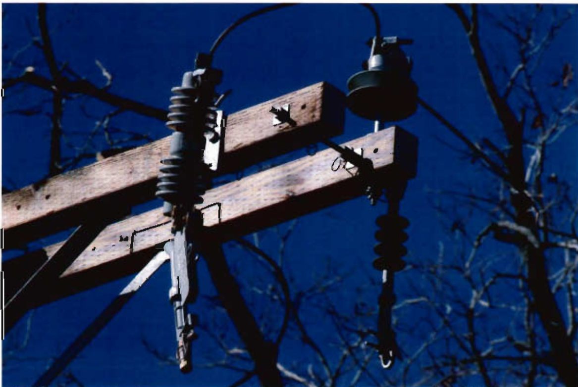
P-KG-172 Close up of hardware on north side of powerpole number 1854107E, facing southwest
