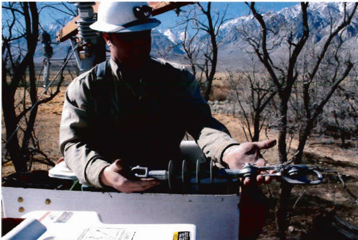
P-KG-269 [redacted] holding hardware after removing from northwest corner of pole number 1854107E
