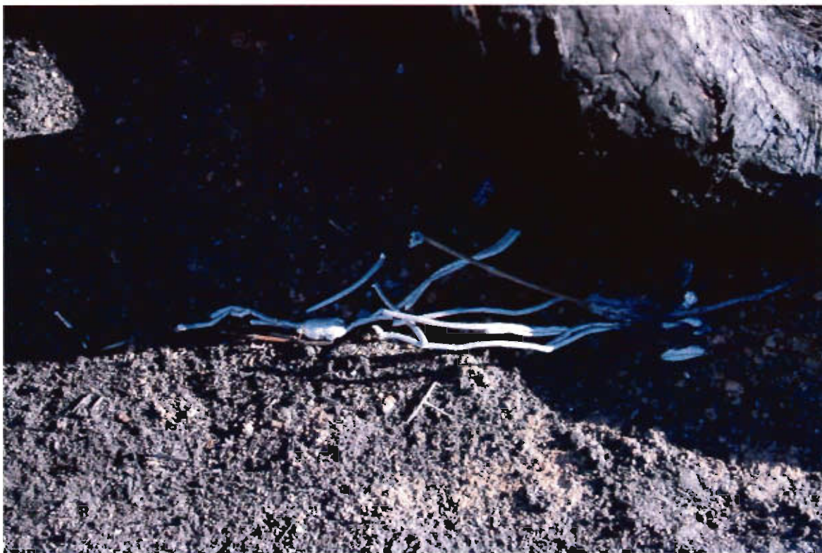
P-KG-244 Close up south power line and small pieces in SOA, facing east
