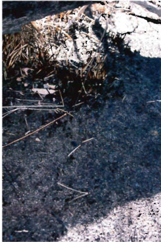
P-KG-161 Close up backing burn indicator, facing southeast, exposed side
