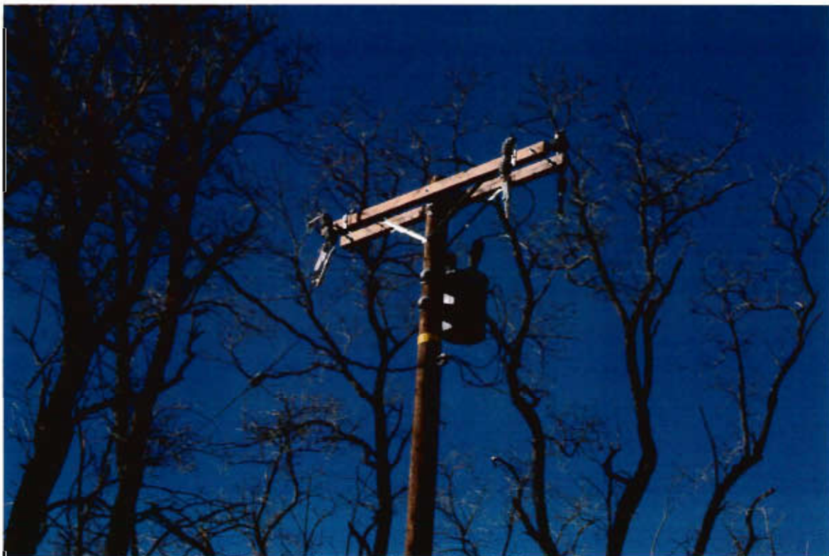
P-KG-170 Powerpole number 1854107E, facing southwest
