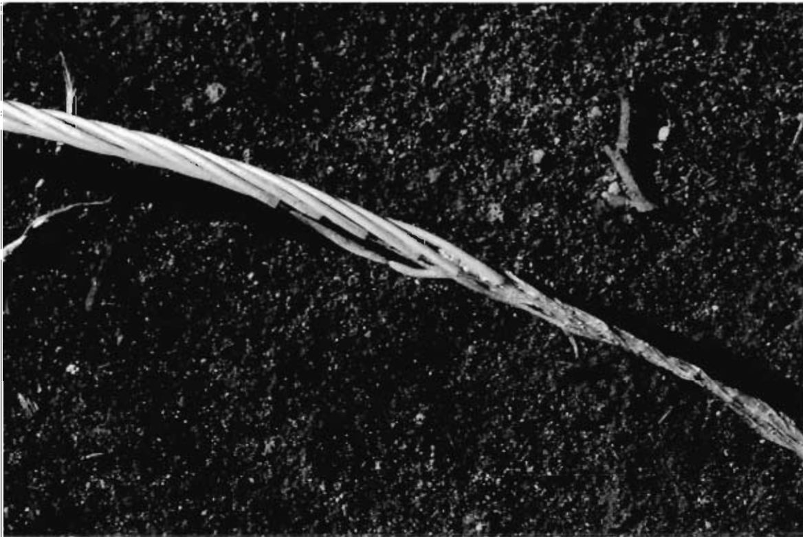
P-KG-374 9d - Close up of power line from east to west
