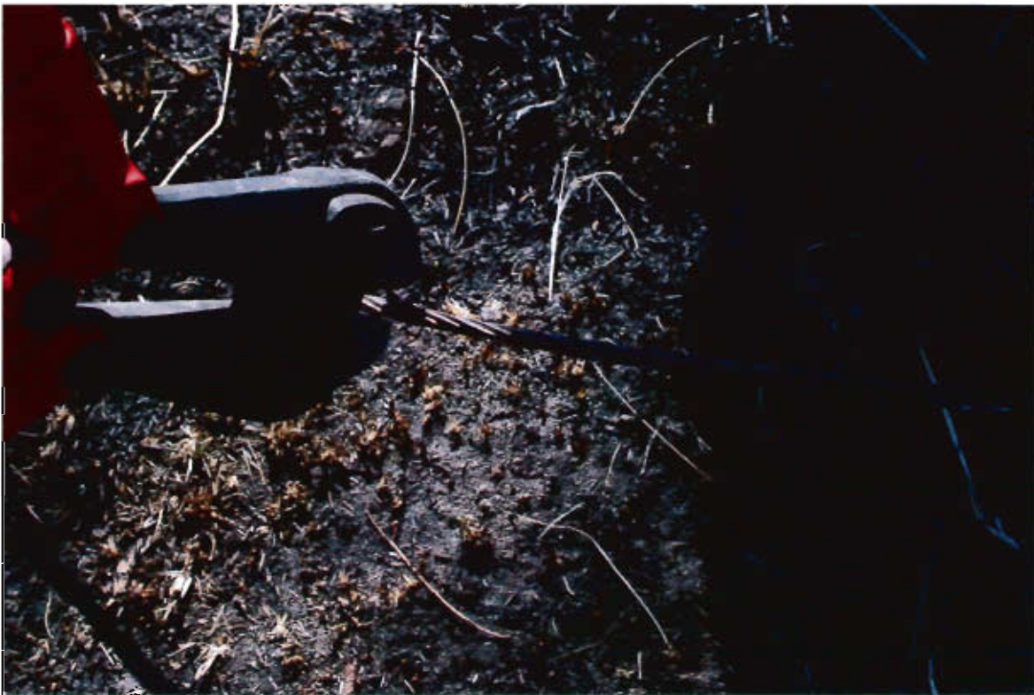
P-KG-318 9a - Cutting power line
