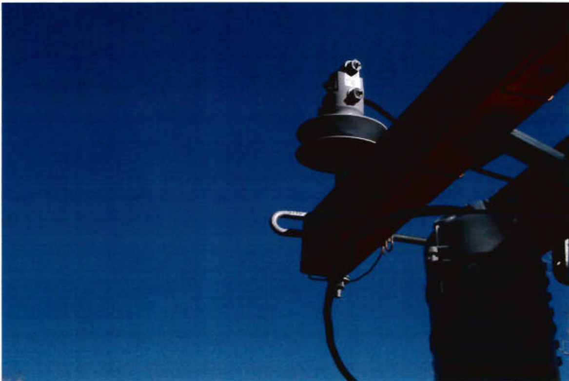
P-KG-280 Northwest corner of pole number 1854107 E after hardware removed, facing northeast
