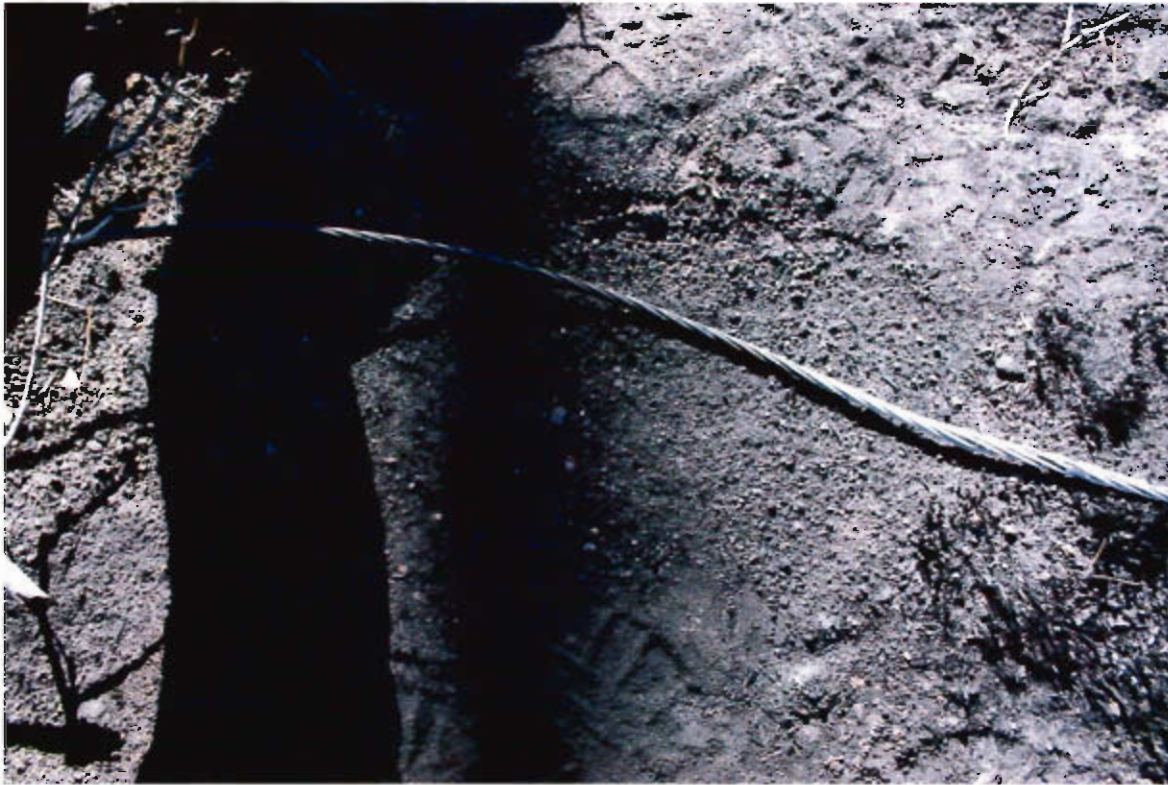
P-KG-305 8c - Power line section close ups from west to east
