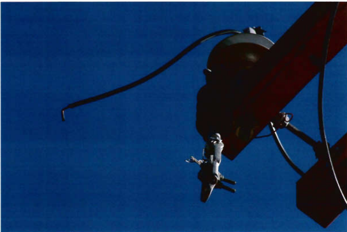
P-KG-258 Close up part of north power line connected to hardware on pole number 1854107E, facing northeast
