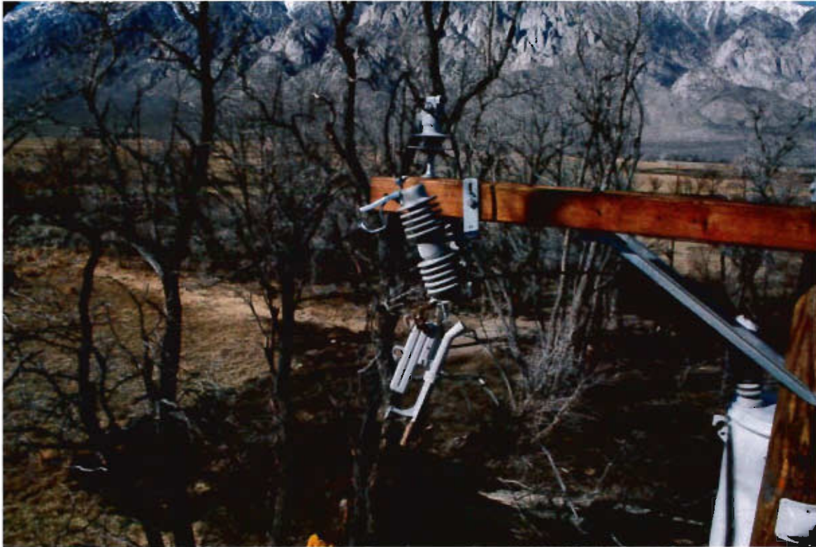
P-KG-271 Close up of hardware on south end of pole number 1854107E from lifted Edison bucket, facing west
