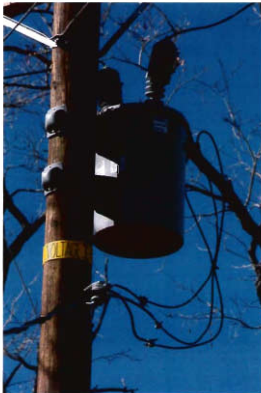
P-KG-174 Close up of transformer and hardware on center of powerpole number 1854107E, facing southwest
