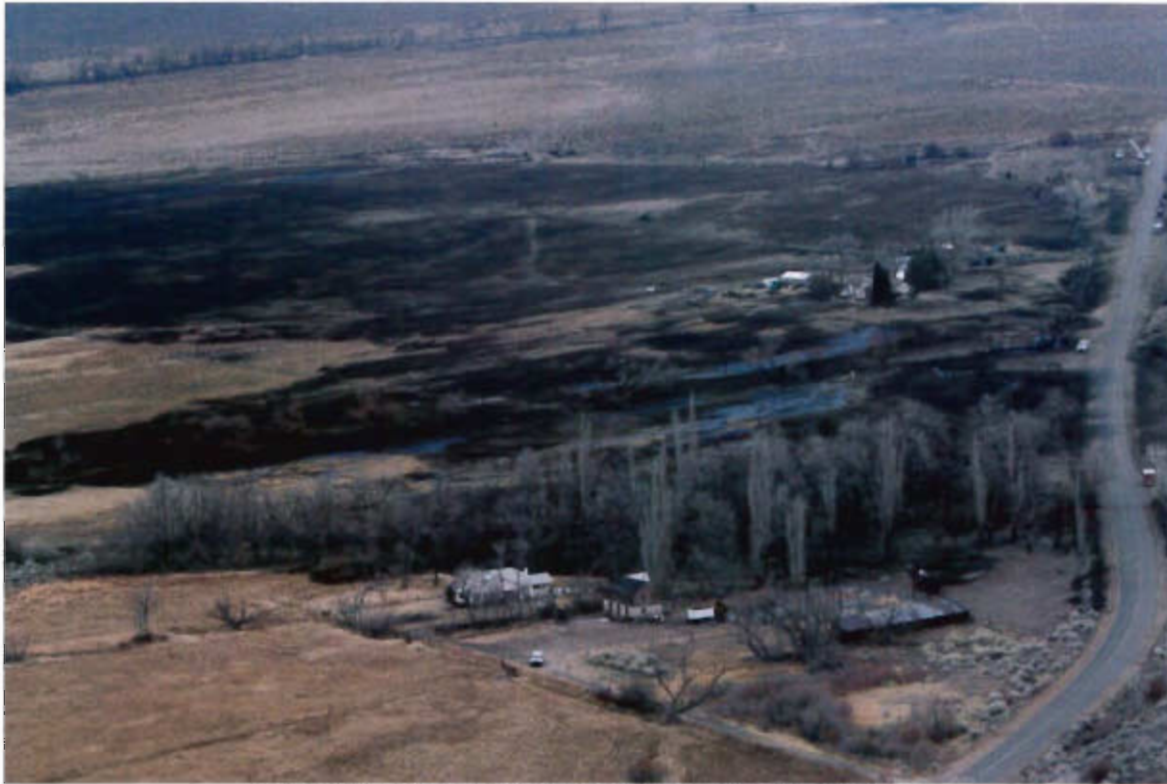
P-KG-011 View towards origin, facing northwest
