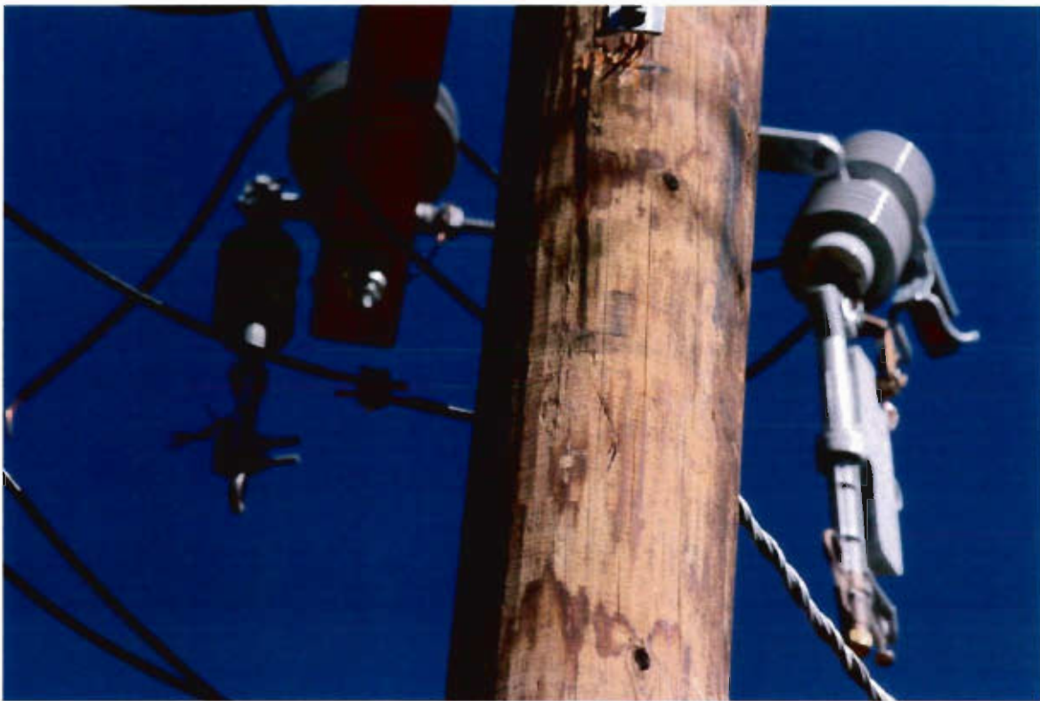
P-KG-175 Close up of hardware on north side of powerpole number 1854107E, facing north
