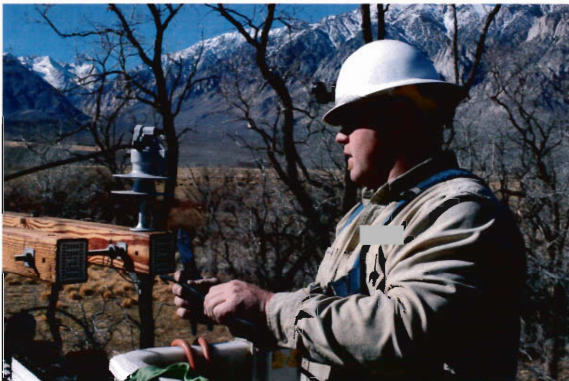
P-KG-270 [redacted] holding hardware after removing from northwest corner of pole number 1854107E
