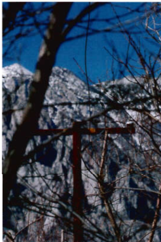
P-KG-200 North powerline, facing west
