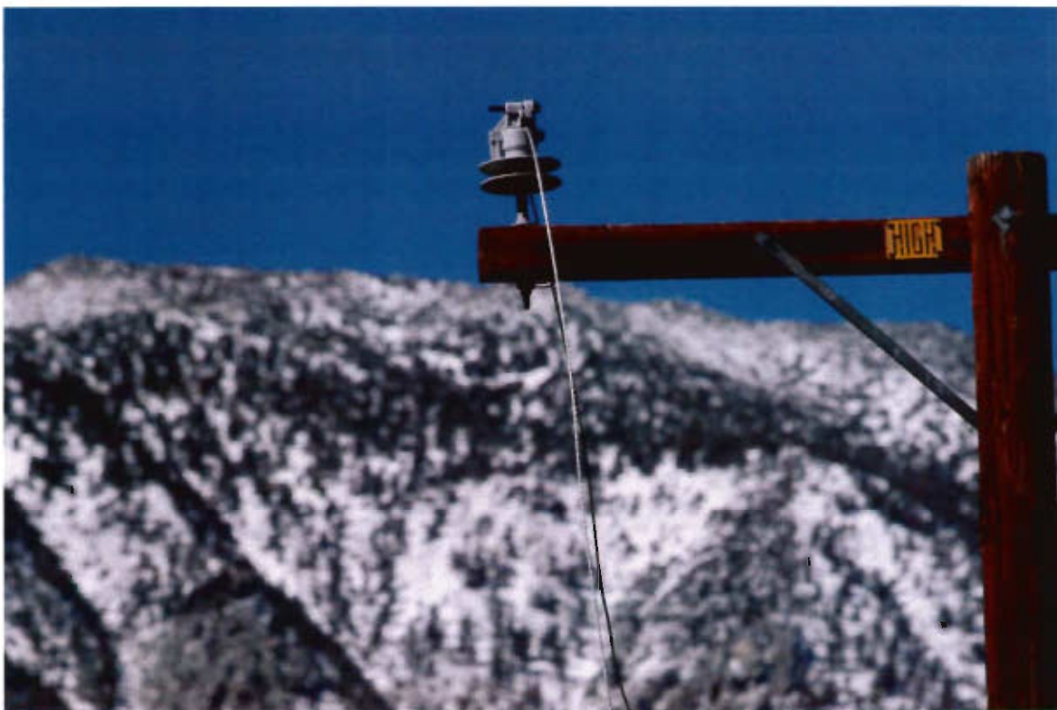
P-KG-188 South powerline attached to powerpole number 1854106E, facing west
