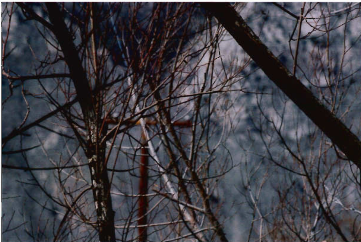
P-KG-202 North powerline, facing west
