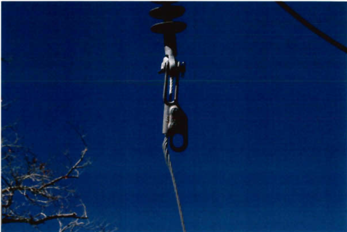
P-KG-273 Close up of hardware on southwest corner of pole number 1854107E from lifted Edison bucket, facing west
