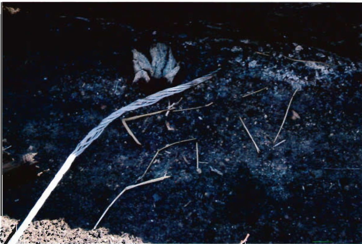
P-KG-250 Close up of south power line in SOA, facing east
