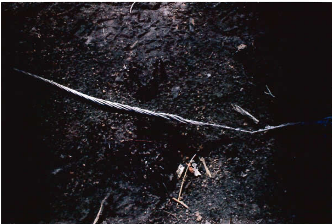
P-KG-304 8c - Power line section close ups from west to east
