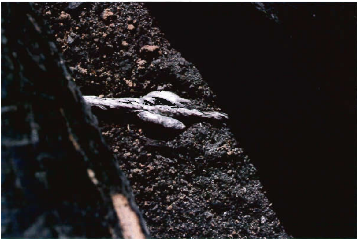
P-KG-350 9c - Power line section close ups from west to east
