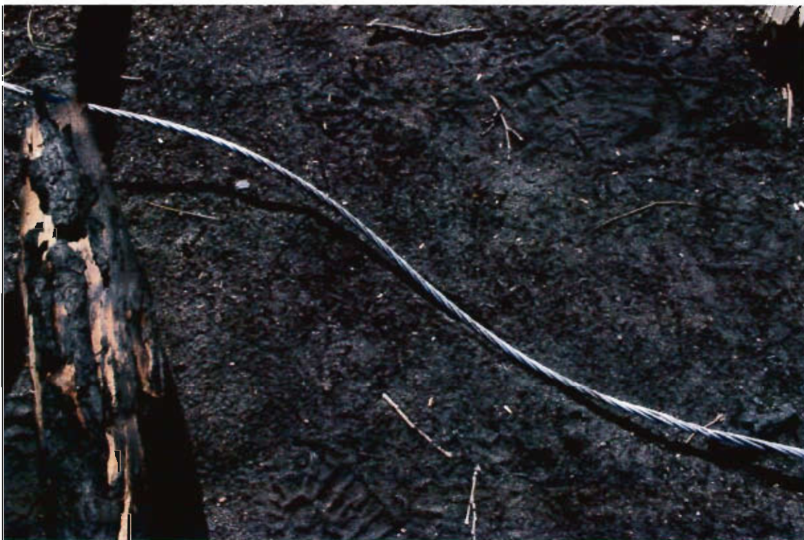
P-KG-334 9b - Power line section close ups from west to east
