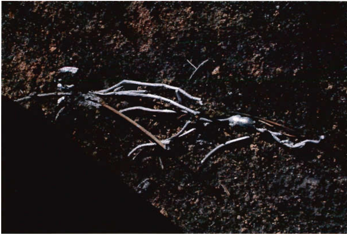
P-KG-349 9c - Power line section close ups from west to east
