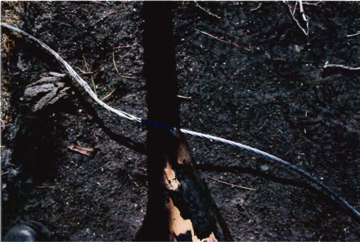
P-KG-335 9b - Power line section close ups from west to east
