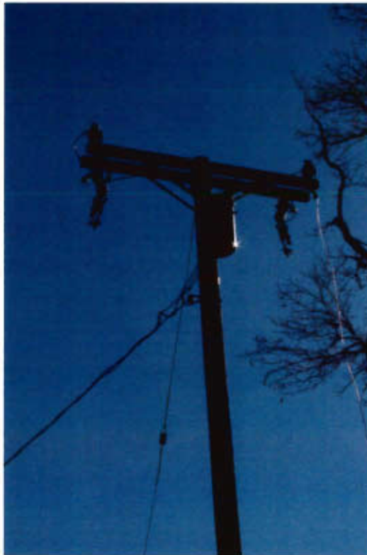
P-KG-169 Powerpole number 1854107E, facing southeast
