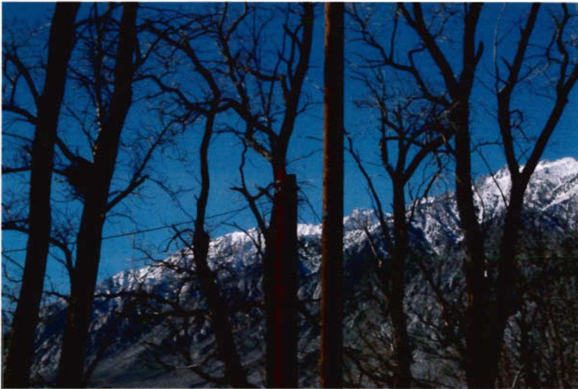
P-KG-171 Powerpole number 1854107E, facing southwest - both powerpoles have same pole number
