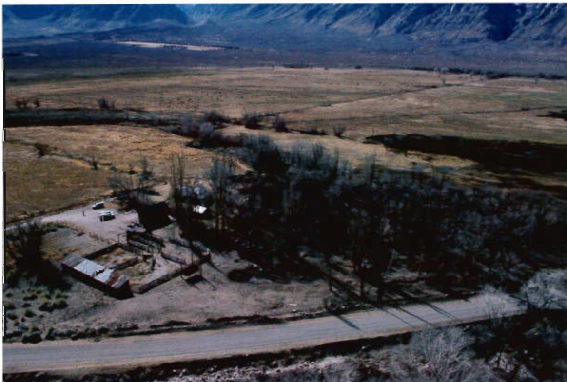
P-KG-230 View towards origin, facing southwest
