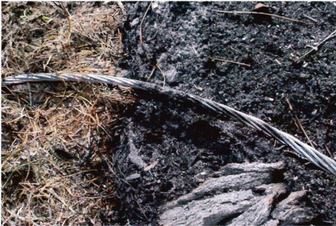
P-KG-337 9b - Power line section close ups from west to east
