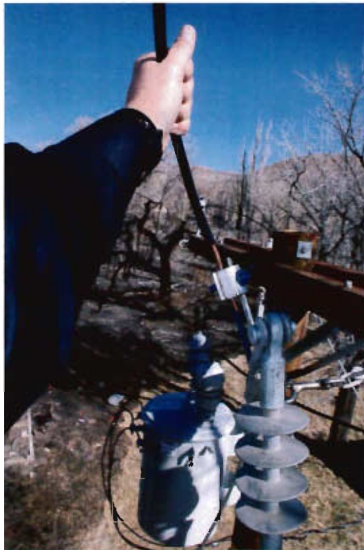
P-KG-278 Close up of hardware from southwest corner of pole number 1854107E after removed via cotter pin connector from end of insulator. Hardware attached to rope line
