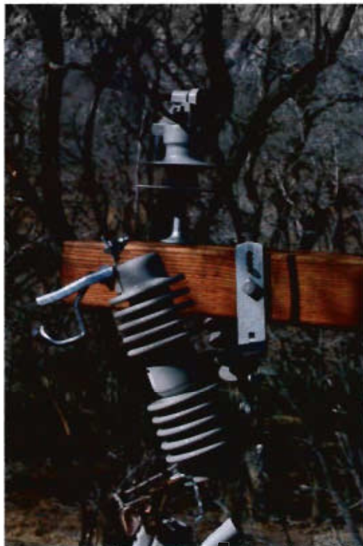
P-KG-272 Close up of hardware on south end of pole number 1854107E from lifted Edison bucket, facing west
