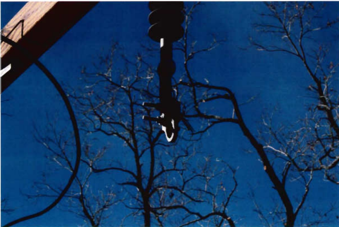
P-KG-266 Close up of hardware with piece of north power line on northwest corner of pole number 1854107E from lifted Edison bucket, facing southwest
