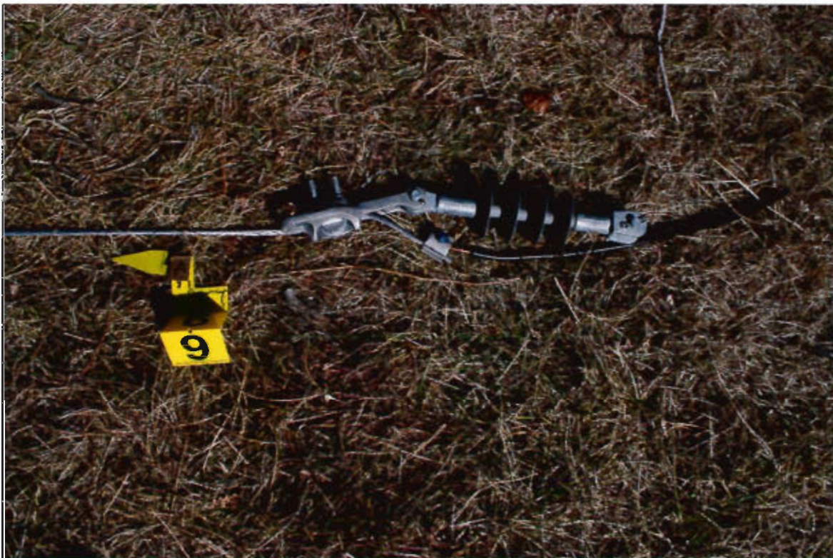
P-KG-316 9a - 12KV deadline poly insulator, wire shoe and jumper wire (protected ground wire - PGW) from south powerline
