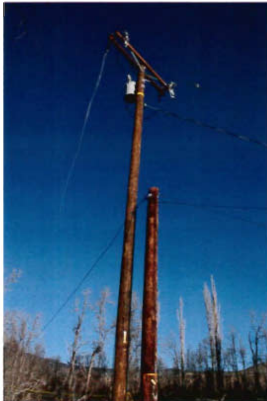
P-KG-038 Power pole east of GOA, number 1854107, facing N
