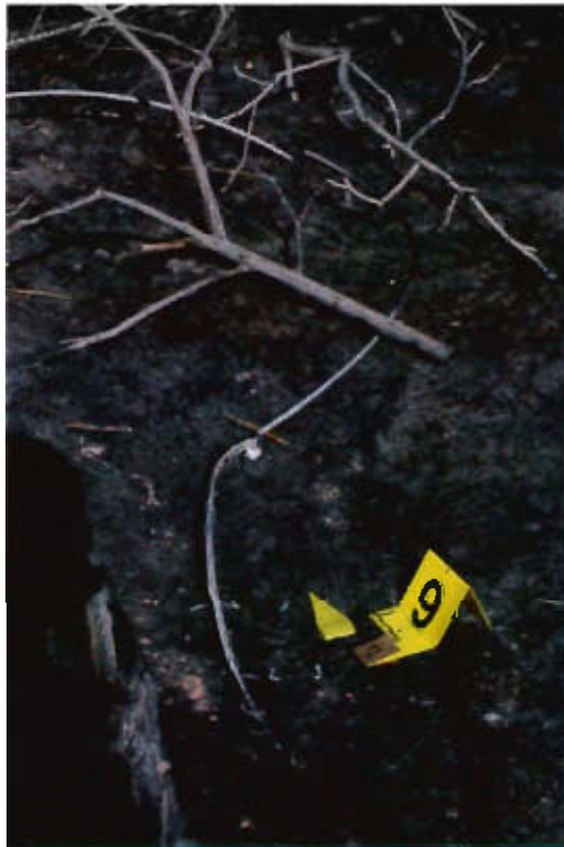
P-KG-368 9d - Power line section after cut
