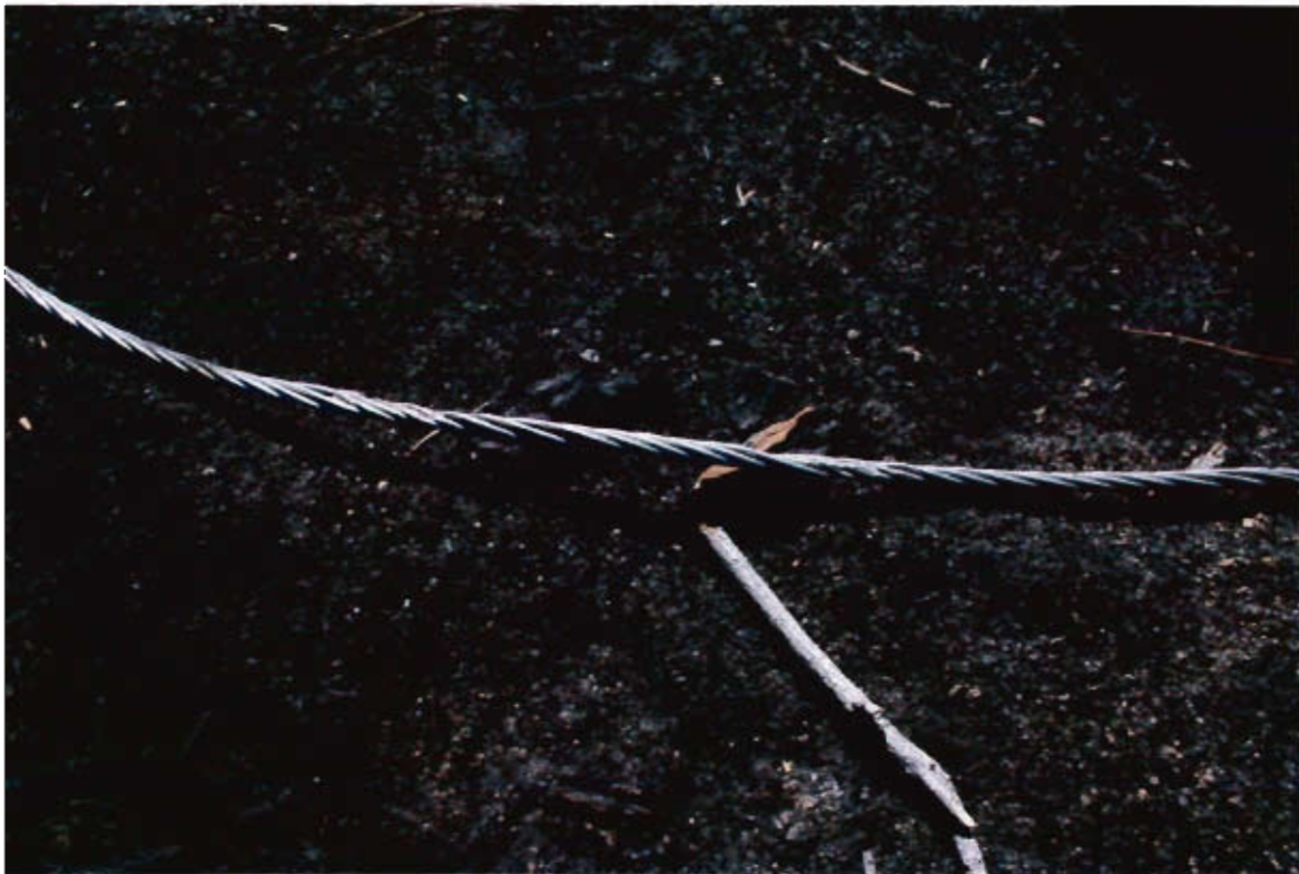
P-KG-333 9b - Power line section close ups from west to east
