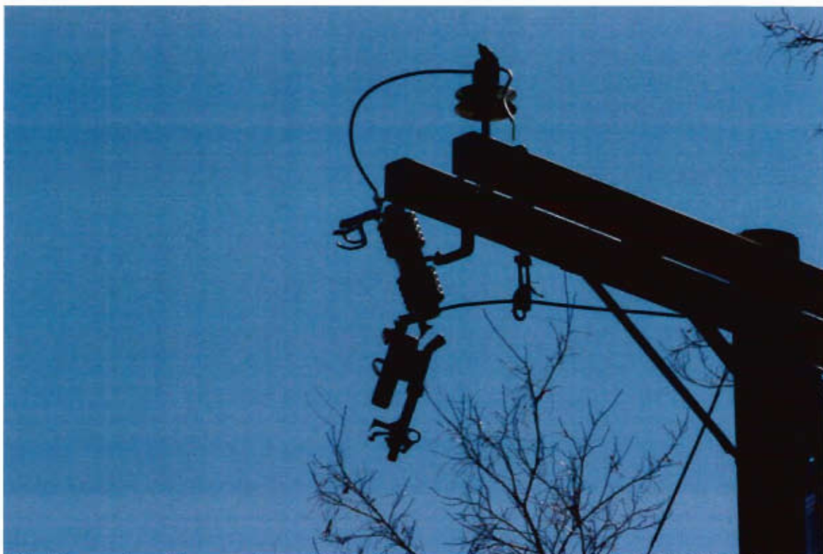
P-KG-189 Piece of north powerline attached to powerpole number 1854107E, facing southeast
