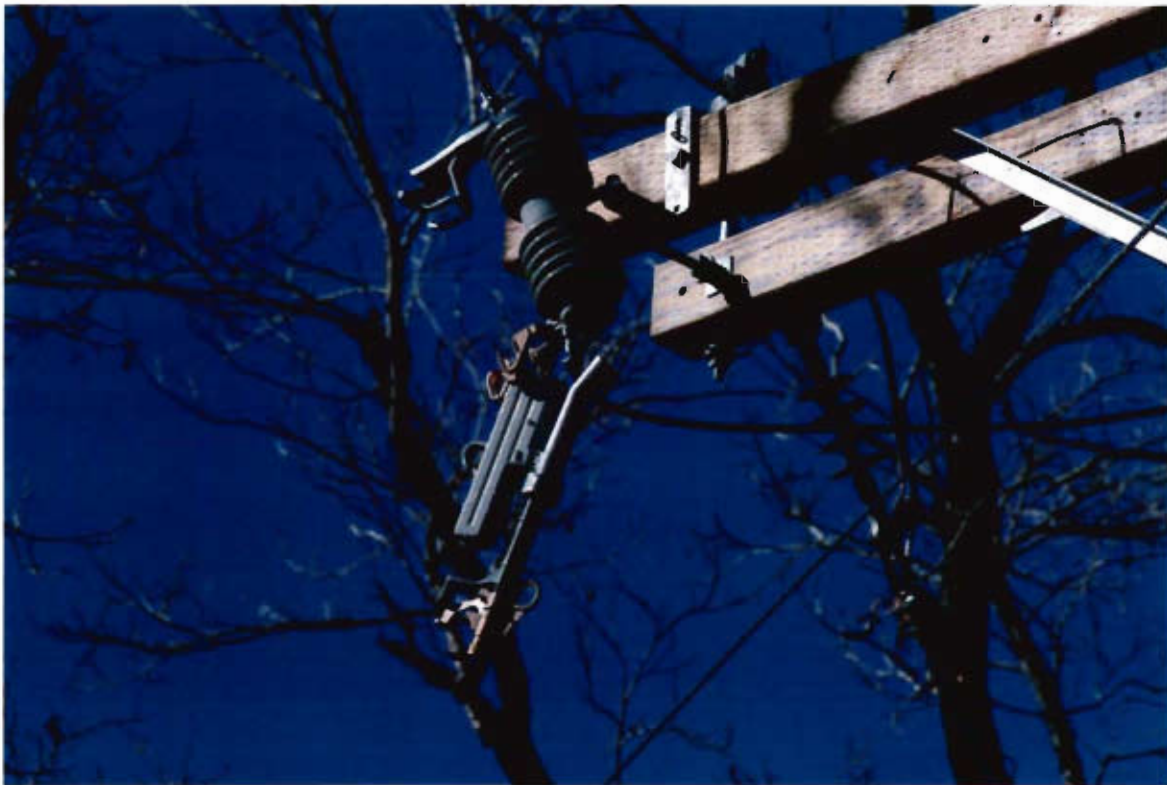
P-KG-173 Close up of hardware on south side of powerpole number 1854107E, facing southwest
