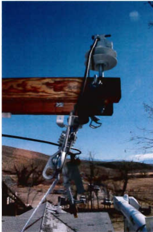
P-KG-277 Close up of hardware on southwest corner of pole number 1854107E from lifted Edison bucket, facing east
