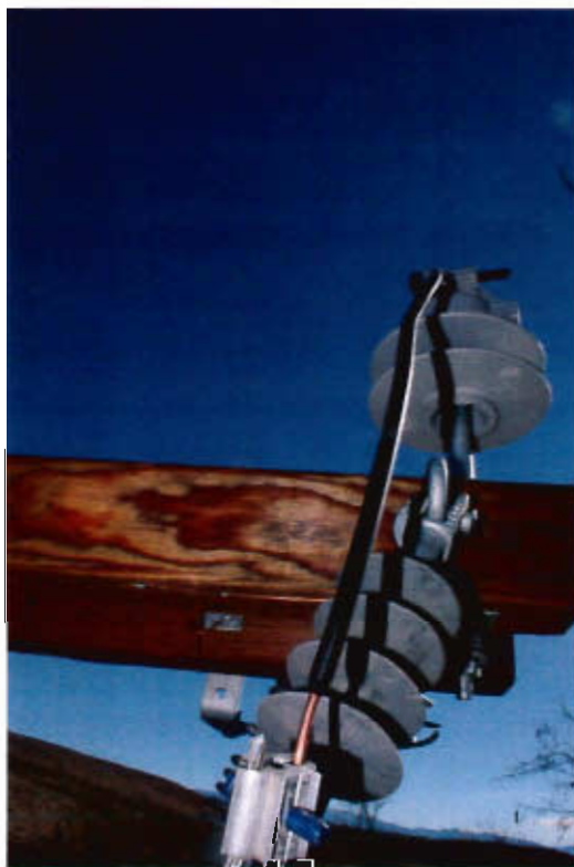
P-KG-276 Close up of hardware on southwest corner of pole number 1854107E lifted Edison bucket, facing east
