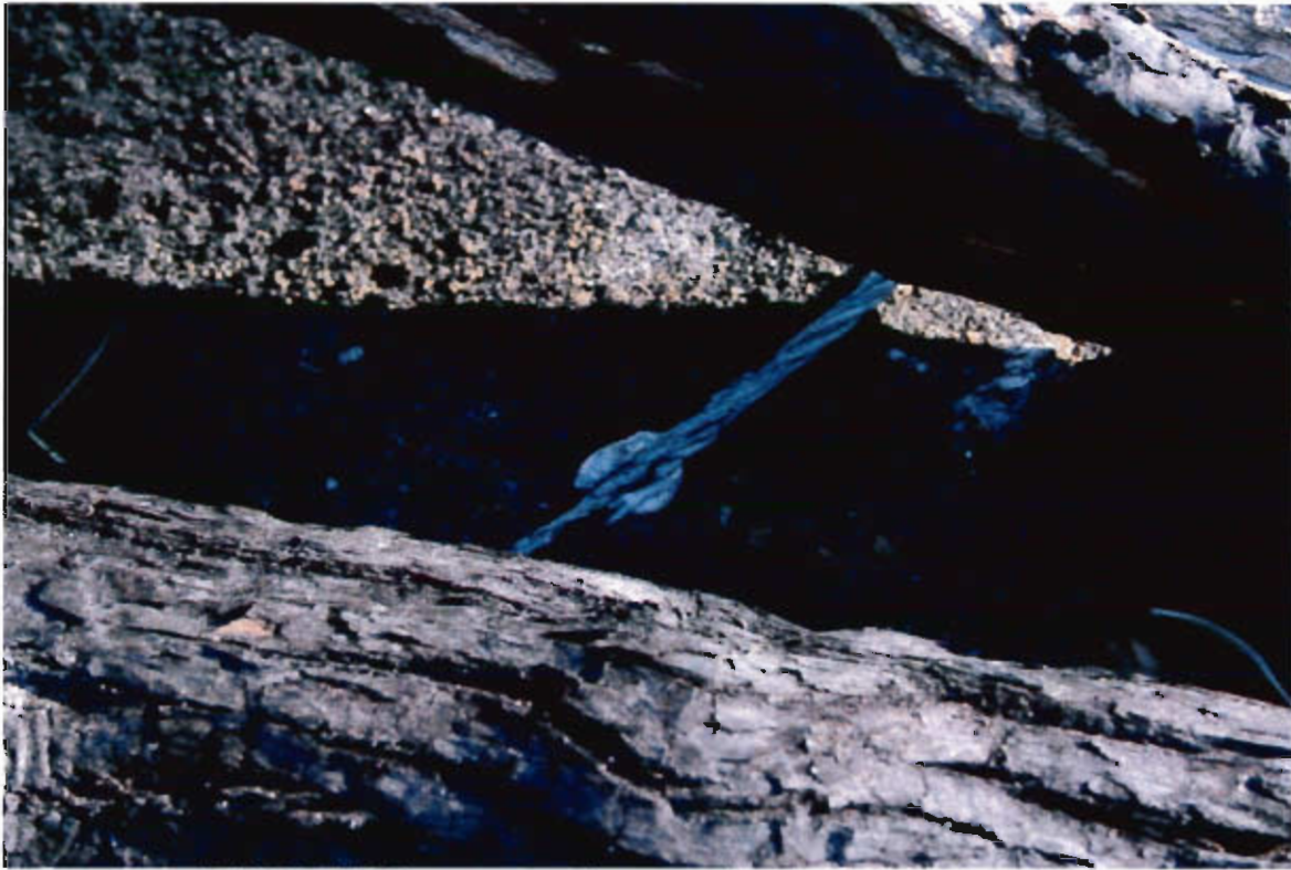
P-KG-247 Close up south power line in SOA, facing east
