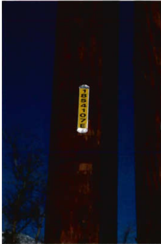
P-KG-039 Close up of power pole number east of GOA, number 1854107, facing N
