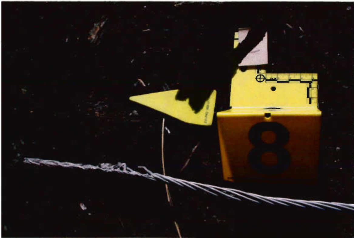
P-KG-297 8c - Power line section close ups from west to east
