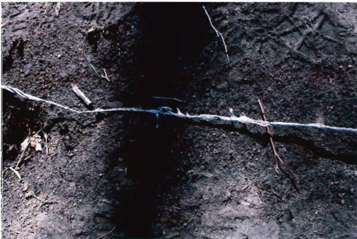
P-KG-302 8c - Power line section close ups from west to east
