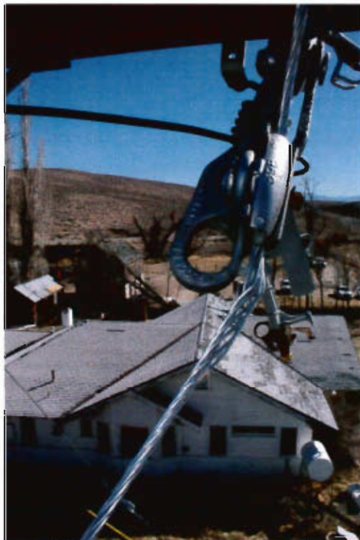
P-KG-274 Close up of wire shoe on southwest corner of pole number 1854107E from lifted Edison bucket, facing east
