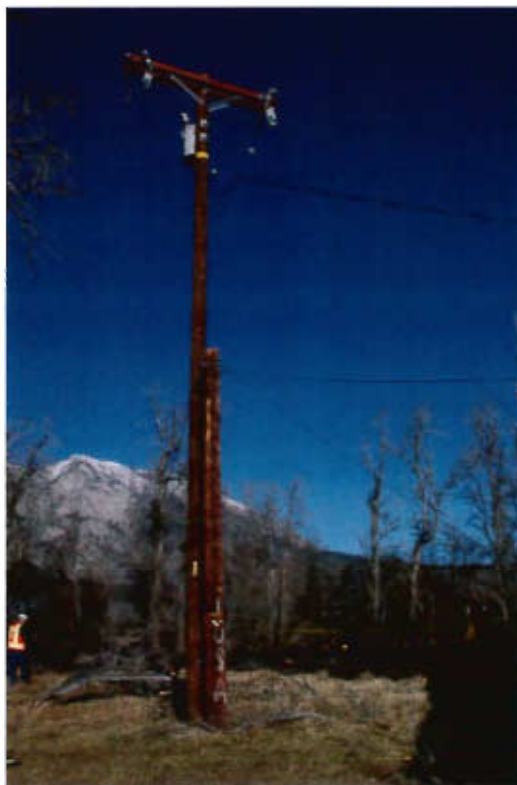
P-KG-040 Power pole east of GOA, number 1854107, facing west
