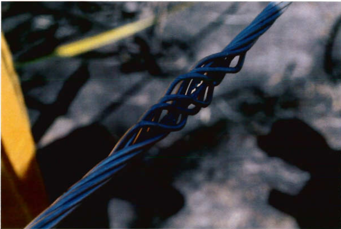
P-KG-293 8b - Close up of damaged wire section
