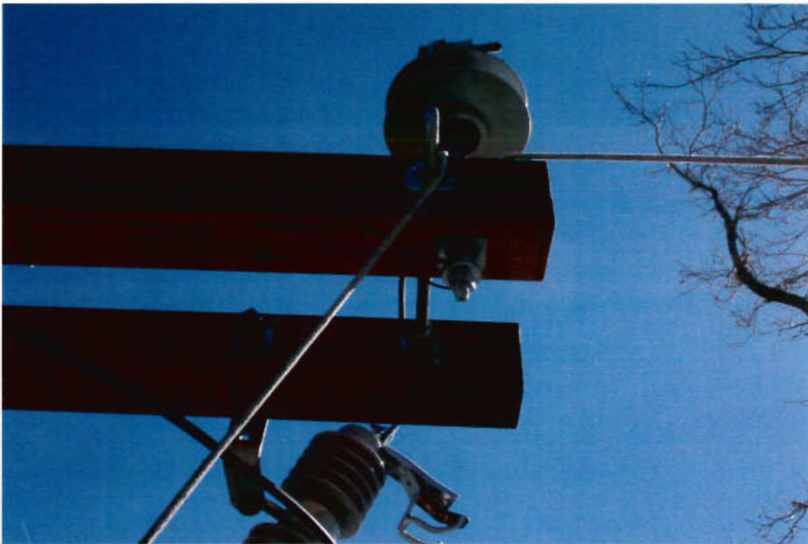
P-KG-281 Southwest corner of pole number 1854107 E after hardware removed, rope line used for lowering hardware, facing east
