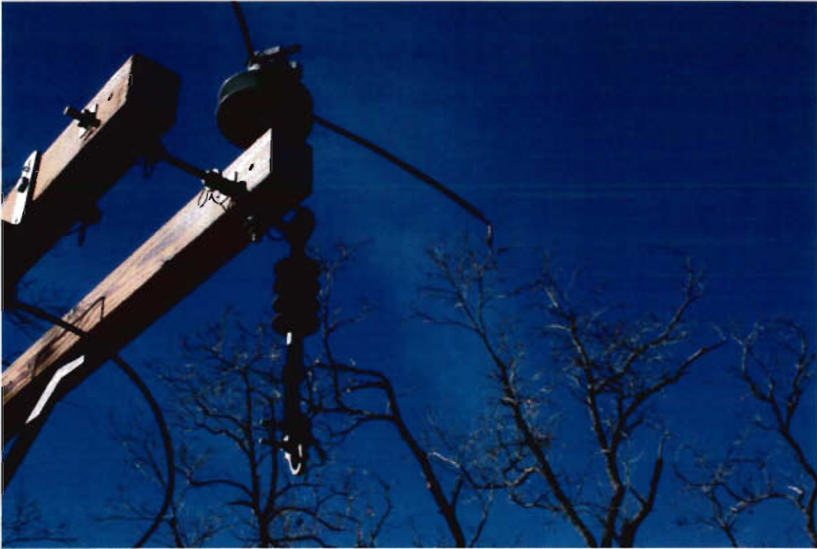
P-KG-265 Close up of hardware on northwest corner of pole number 1854107E from lifted Edison bucket, facing southwest
