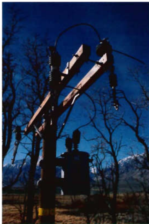
P-KG-264 Close up top of pole number 1854107E from lifted Edison bucket, facing southwest
