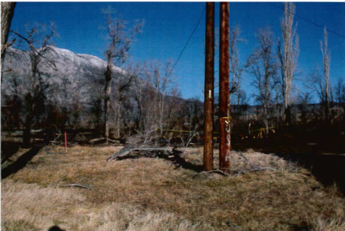
P-KG-036 Overall facing northwest towards GOA
