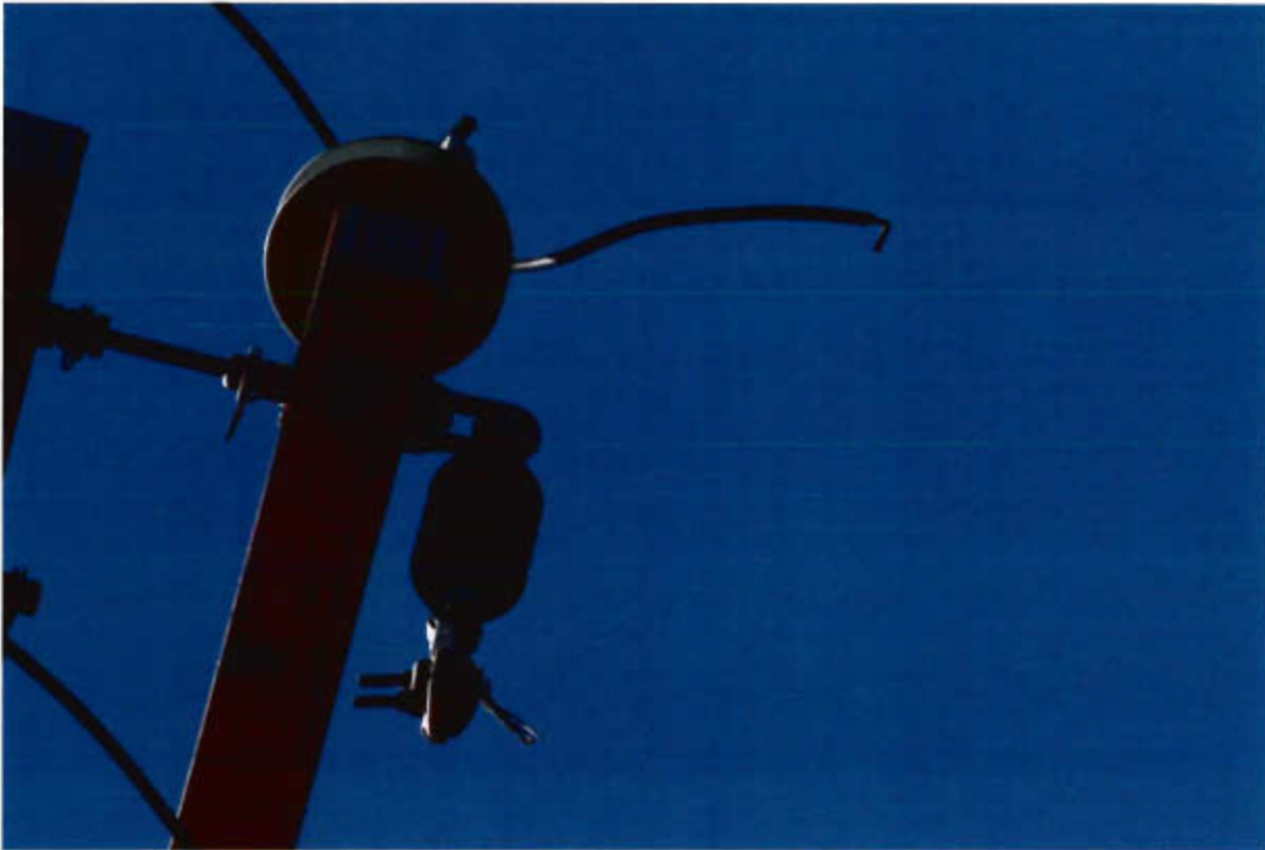
P-KG-259 Close up part of north power line connected to hardware on pole number 1854107E, facing south
