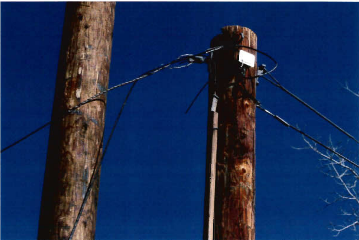
P-KG-178 Close up of hardware of powerpole number 1854107E, facing north - both powerpoles have the same pole number
