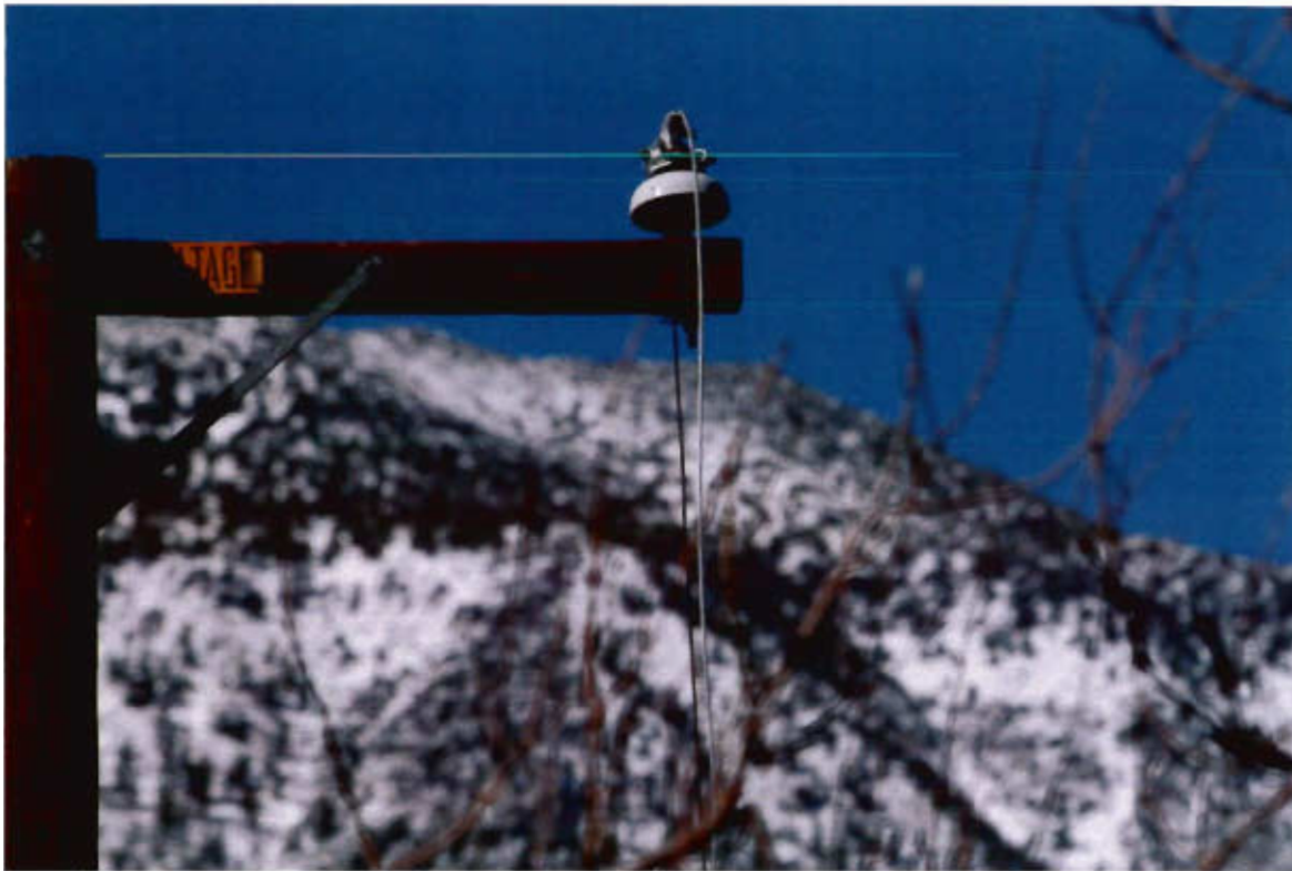
P-KG-203 North powerline attached to powerpole number 1854106E, facing west
