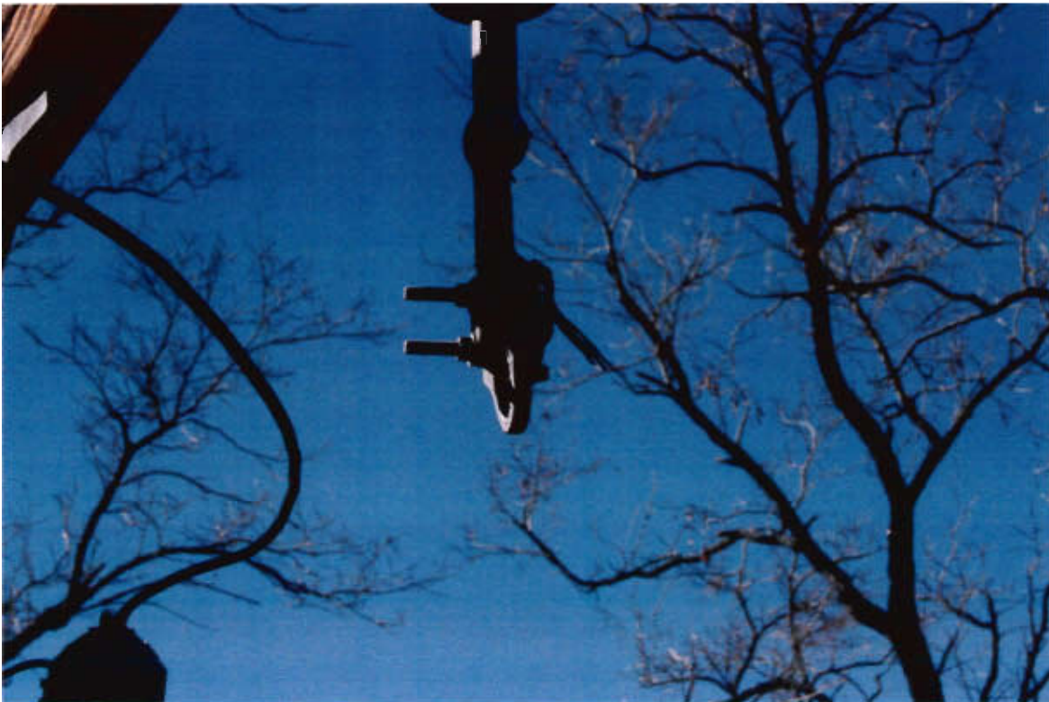
P-KG-268 Close up of hardware with piece of north power line on northwest corner of pole number 1854107E from lifted Edison bucket, facing southwest
