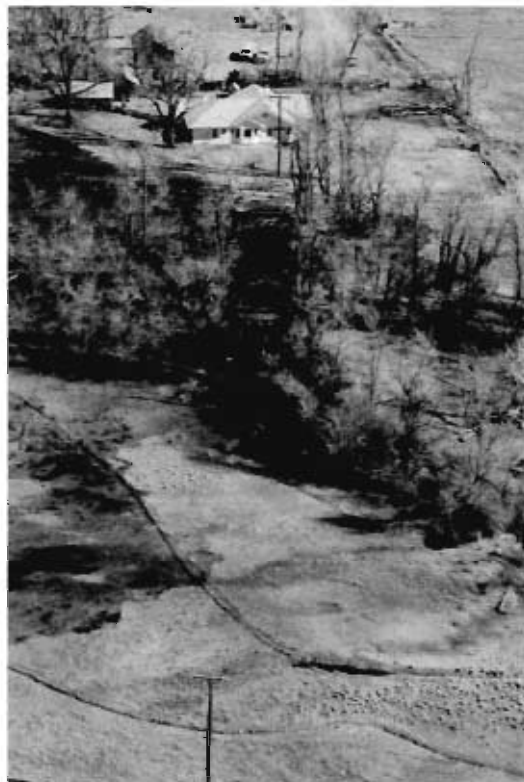
P-KG-222 Overview of power lines running east and west, facing east towards origin
