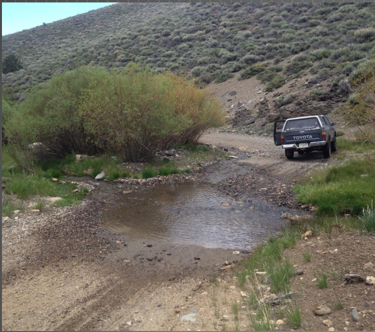
Washed out crossing
