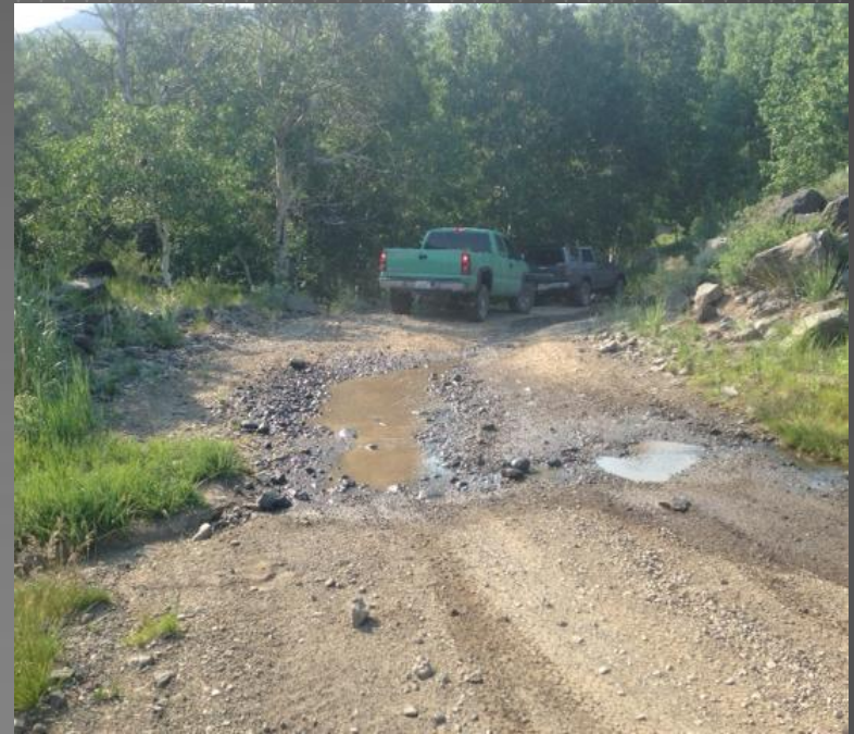
Repaired crossing designed for driveability, drainage, and creek flow
