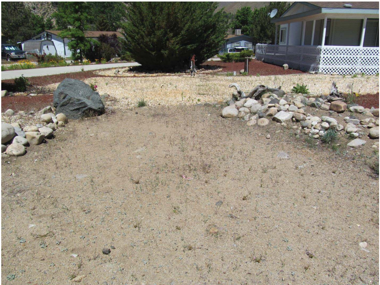
Figure 3. Location of the new Cold Well in the foreground (pink flagging) and location of the old Cold Well in the background.
