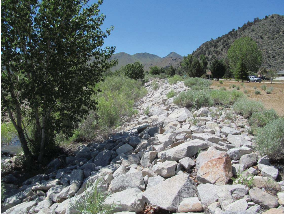
Figure 6. Rip rap covering the eastern edge of the terrace.
